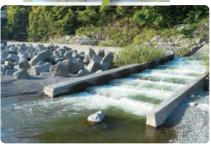
Fishway that was constructed in Toshima Dam
